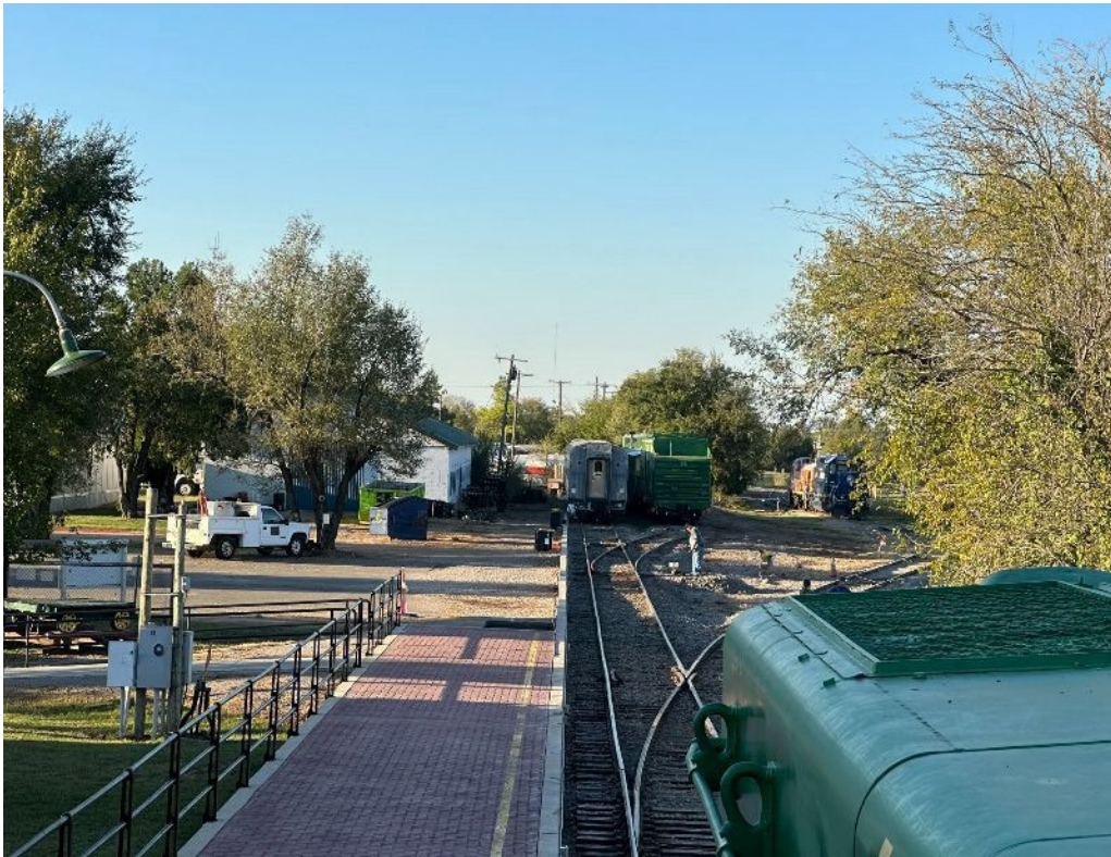
Looking north from the platform shows the new siding off the house track and the extension of the house track.
