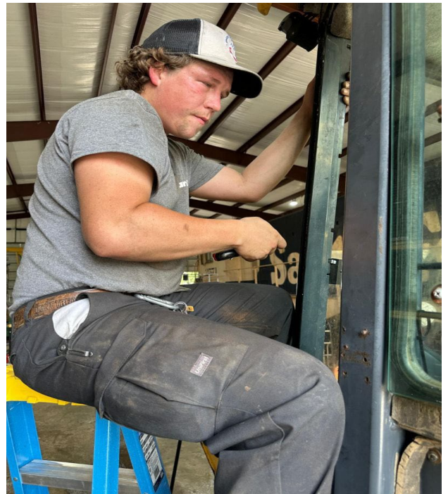
Volunteer Dustin Donaldson works on cleaning the side on the backhoe cab so a new window can be installed.
