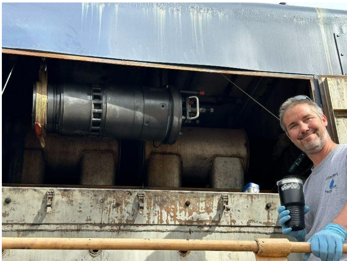
Volunteer and Vice President John Nave, along with Greg Hall and Eric Dilbeck get ready to install a rebuilt power assembly into our Santa Fe CF-7.
