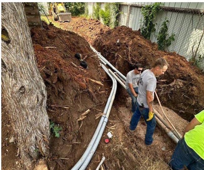
Work on our new electrical service continues progress. Above left, Workers run new conduit and place a pull box behind Anne's office. Above right, new panels are in place and conduit is being backfilled.
