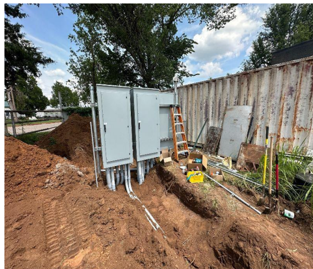
Work on our new electrical service continues progress. Above left, Workers run new conduit and place a pull box behind Anne's office. Above right, new panels are in place and conduit is being backfilled.
