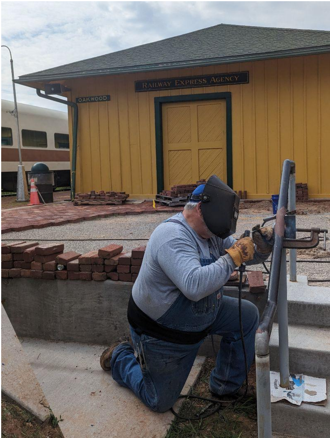
Volunteer Steve Foust welds up a hand rail on the new Oakwood patio assisted by Natalie Lawson.
